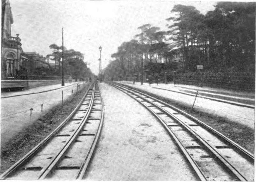
TRACK-CONSTRUCTION WORK IN BOURNEMOUTH, ENGLAND
